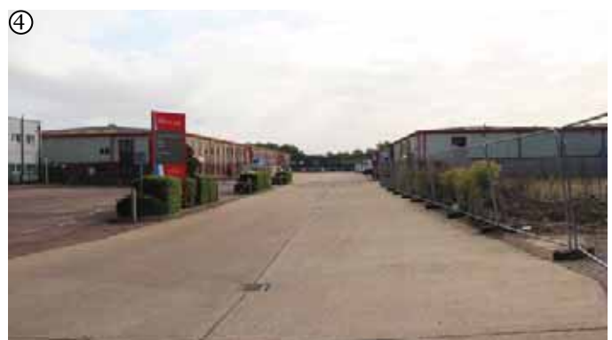
Centrally located internal access road aligned by parking areas and large rectilinear industrial unit
