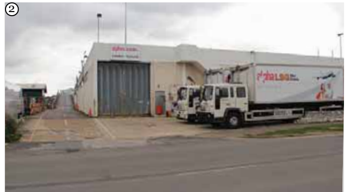
Servicing area and access to Manor Place's rooftop parking, Faraday Road
