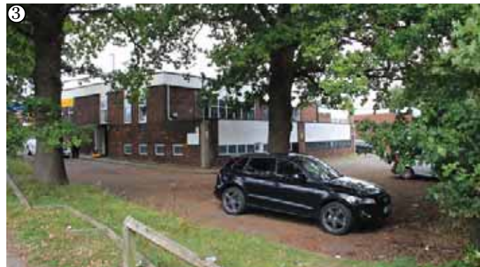
Parking area to the rear of retail units - drop in site levels towards Crawter's Brook
