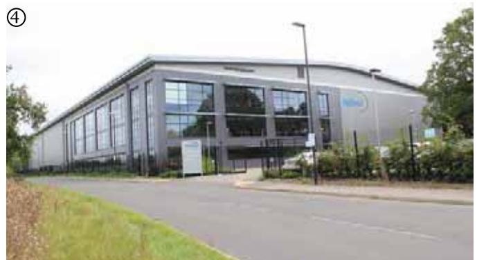
Welland industrial unit located to the south of Hydehurst Lane
