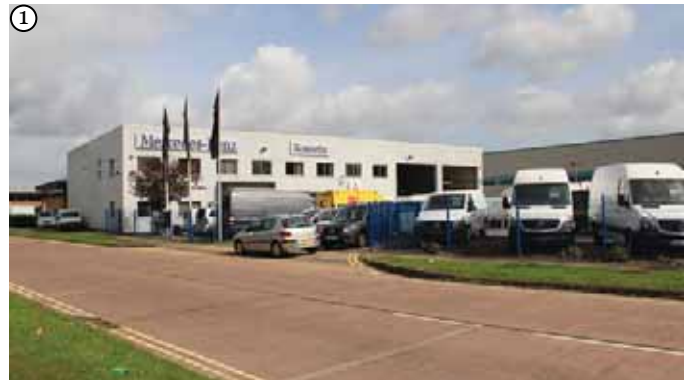
Existing access Newton Road
