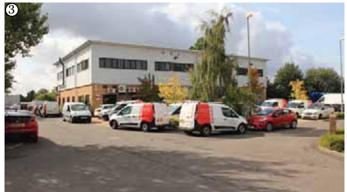
Inaccessible parking area
