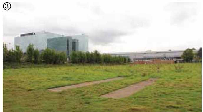
View of site from north western corner
