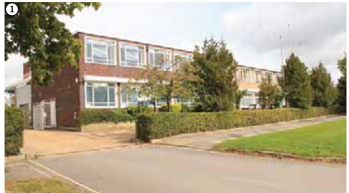
Durand House, existing access, building set back from street frontage via parking area
