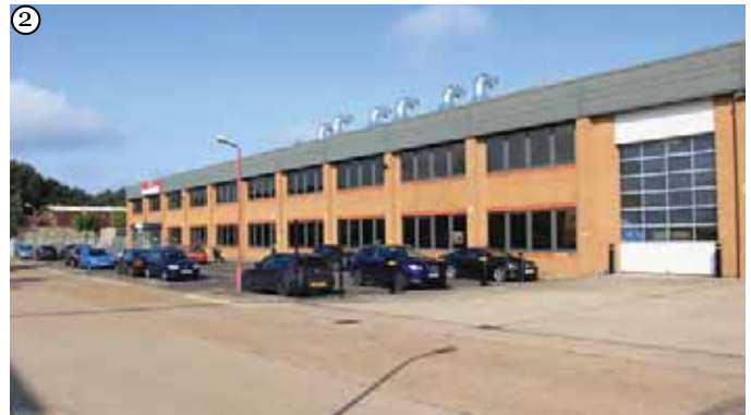
Large rectilinear industrial units
