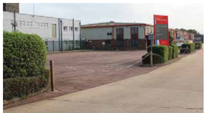
2) Unused car park (as existing, September 2017)
