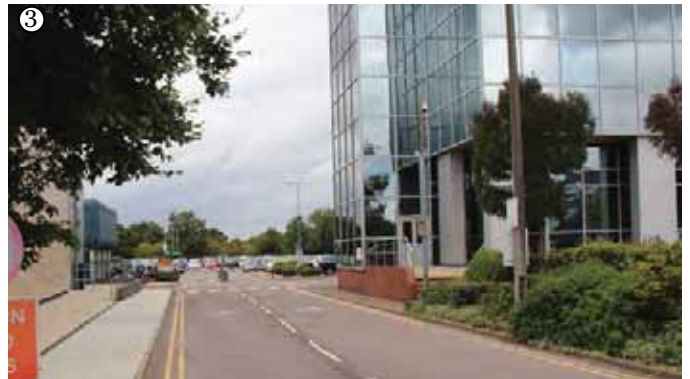
Existing access to Astaral Towers car parking area
