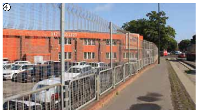
View into site from Gatwick Road
