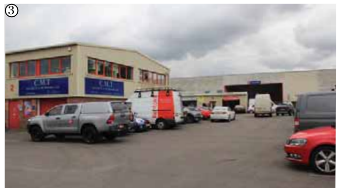
Existing servicing and parking area - large scale industrial unit (background) to the eastern boundary
