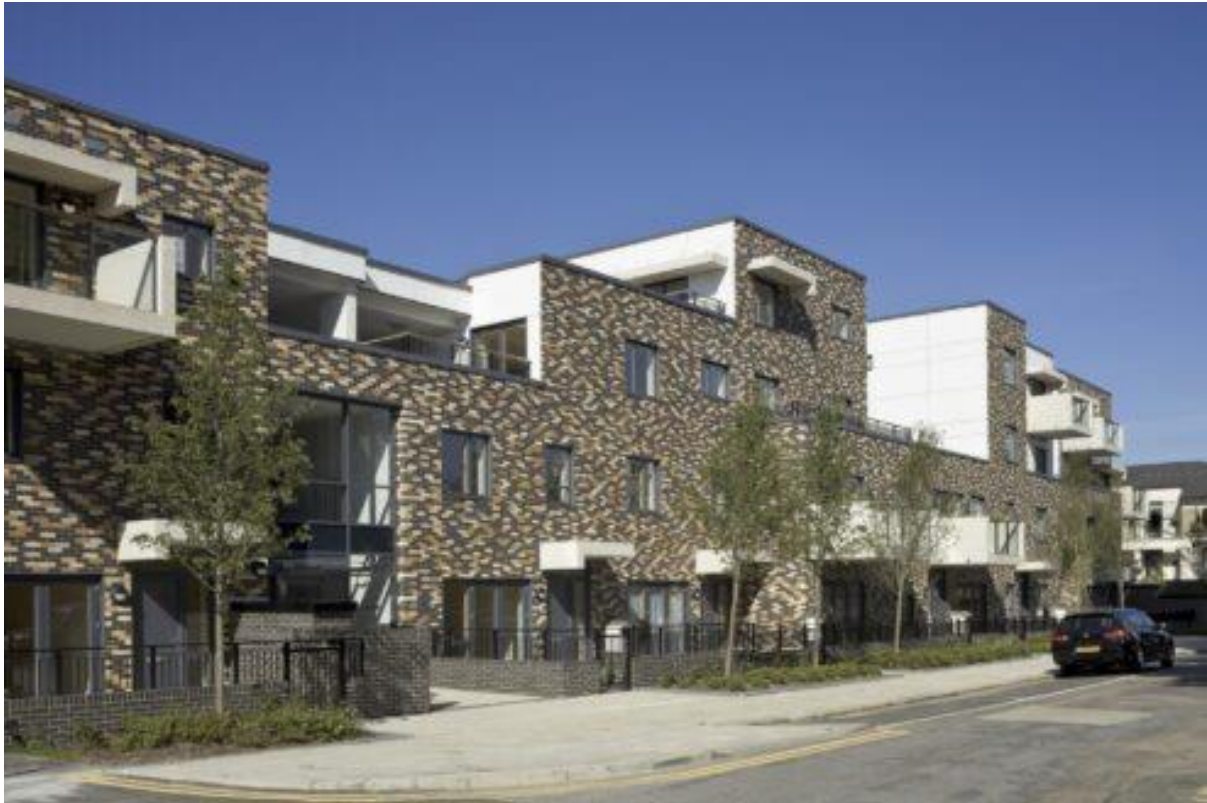
Terraces at upper levels which allow for alternative, useable private outdoor space to be located for top level duplex dwellings.
