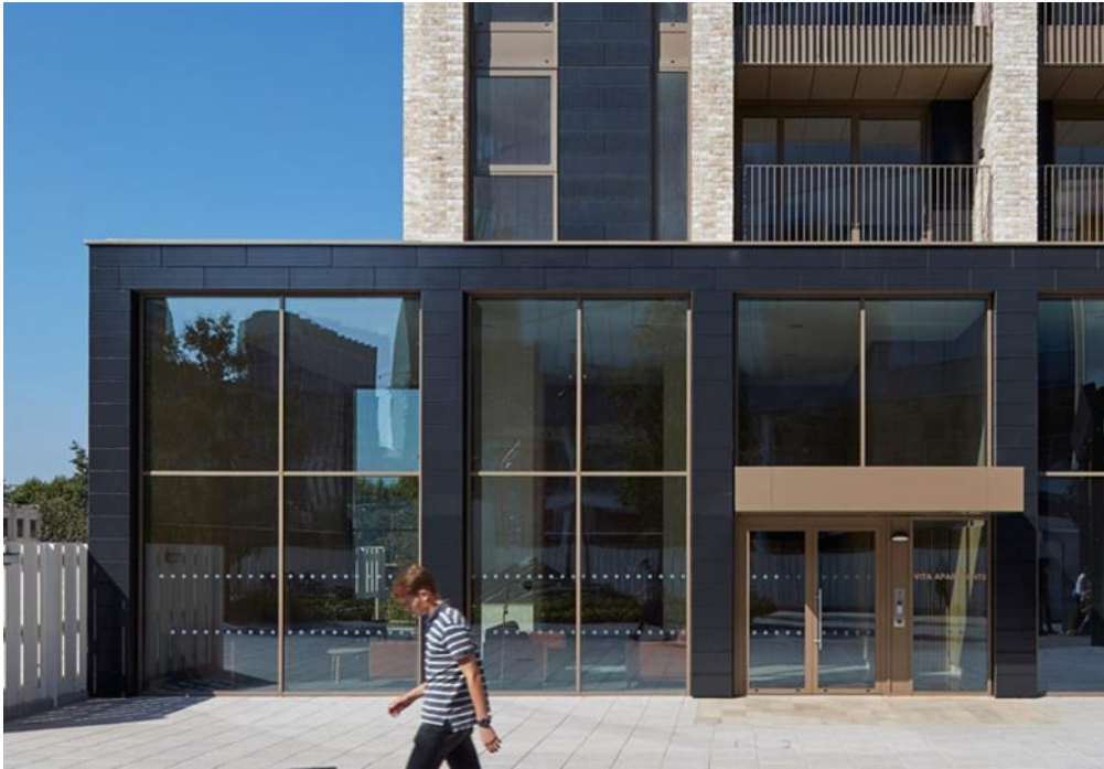
(Above) Vita apartments lobby, Ruskin Square Croydon
