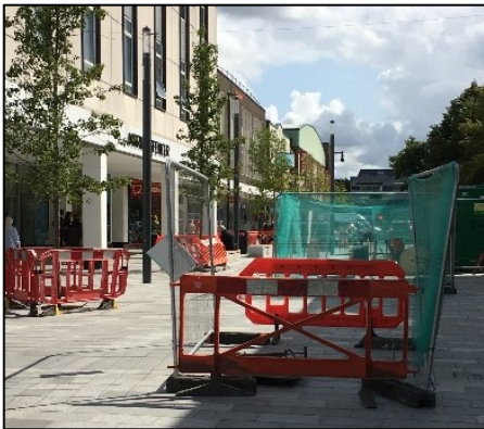
Figure 4.9 | Works ongoing at Queensway
