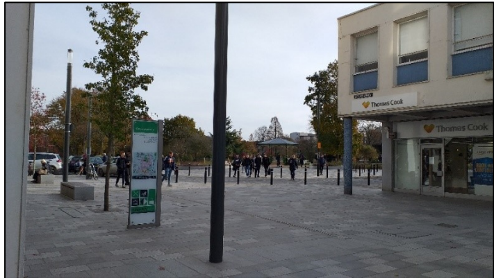
Figure 4.10 | Completed works at Queensway
