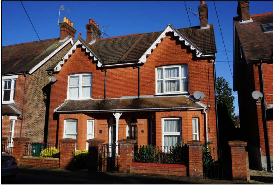
Fig. 14: Projecting porch with slate tiled roof and period detailing. Note also the low level boundary brick wall with capped piers and railings.
