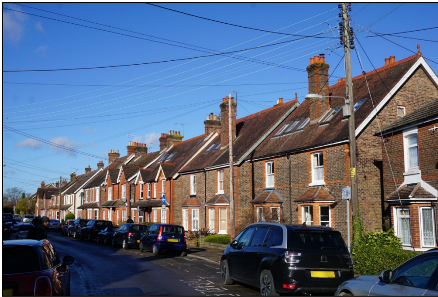
Fig. 13: Ground floor bay windows with lead roll ridges, upper floor sash windows with edge detailing, Hazelwick Road.
