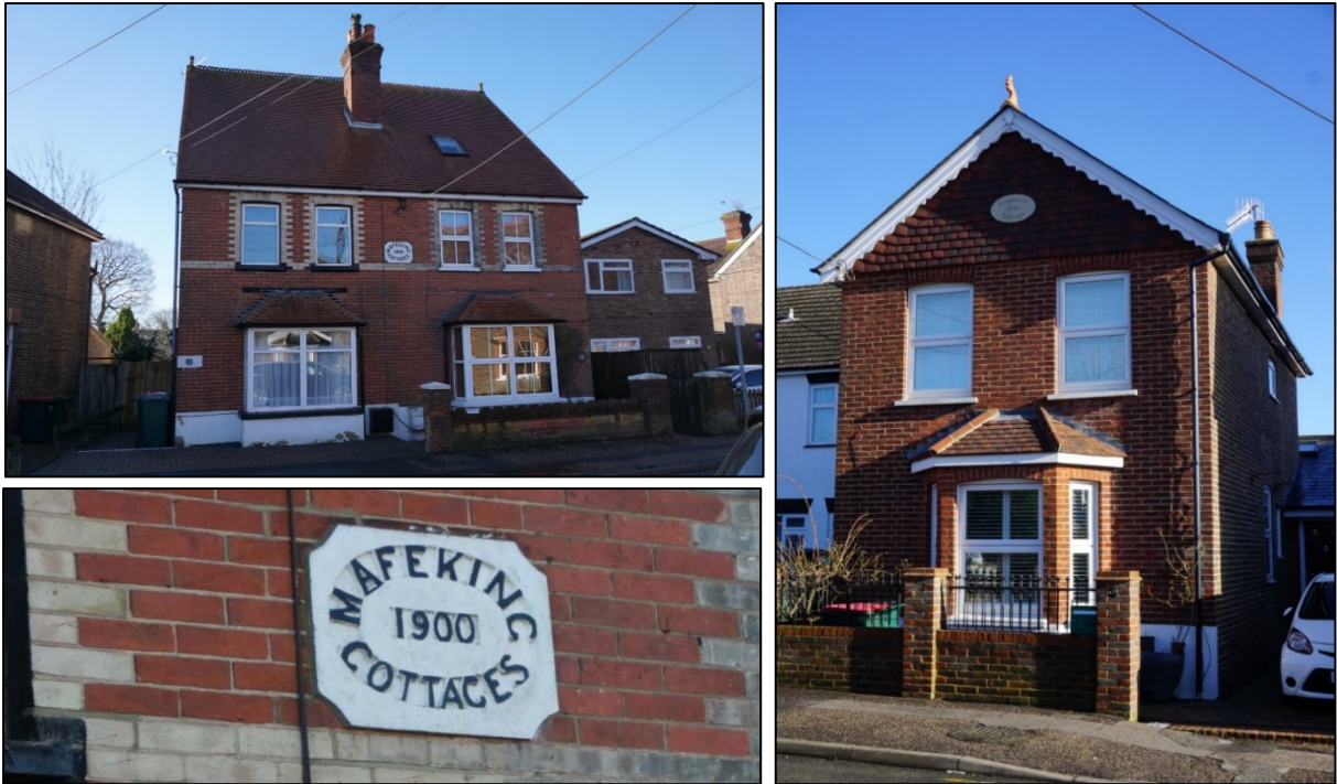
Fig. 11: Several buildings retain interesting period features, including name and date plaques (above left), decorative barge boards, finials and hung tiles (above right). Both 'Mafeking Cottages' and 'Ladysmith Terrace' commemorate the 1899-1900 siege and relief of these South African towns during the Second Boer War.
