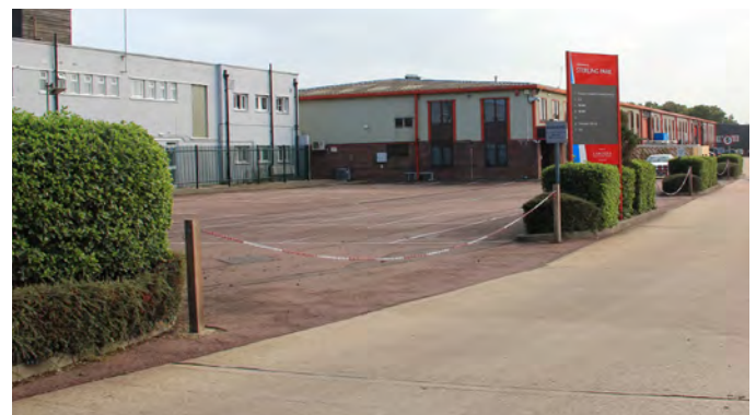
2) Unused car park (as existing, September 2017)
