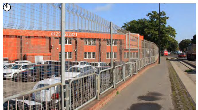
View into site from Gatwick Road
