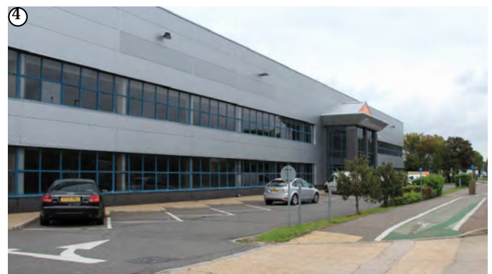
Building frontage set back behind surface parking area
