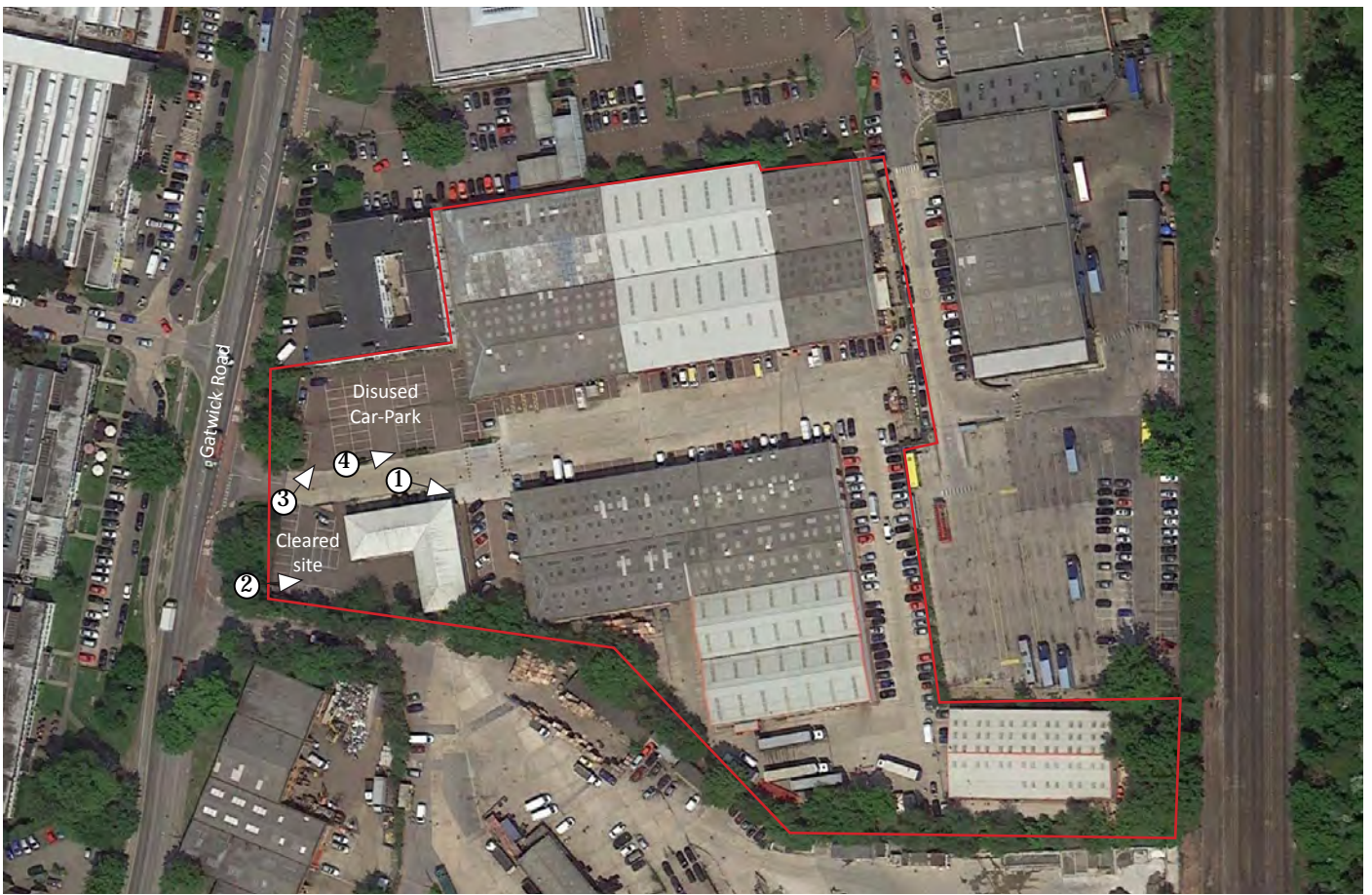
Aerial (Google Earth 2013)
