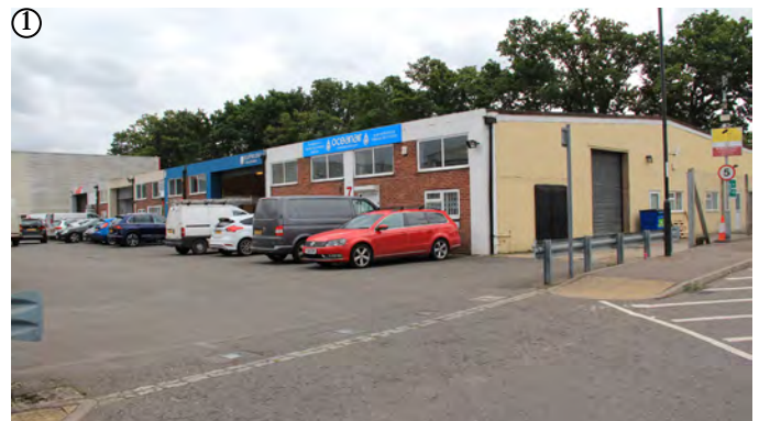
Existing industrial units
