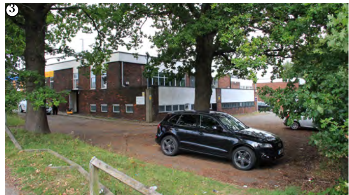
Parking area to the rear of retail units - drop in site levels towards Crawter's Brook
