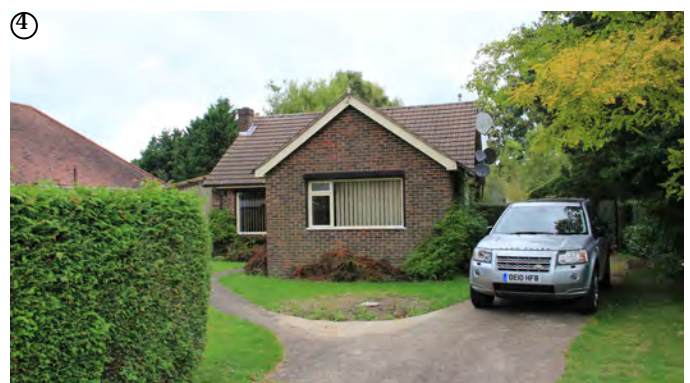
Single storey dwelling Tushmore Lane
