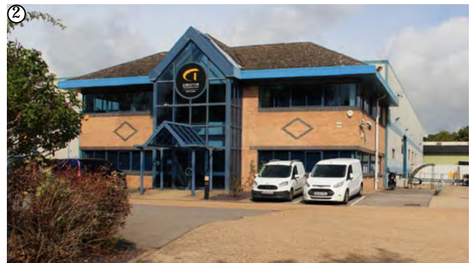
2-3 storey equivalent industrial building with ancillary office space
