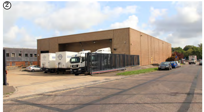
Servicing area and access, Napier Way
