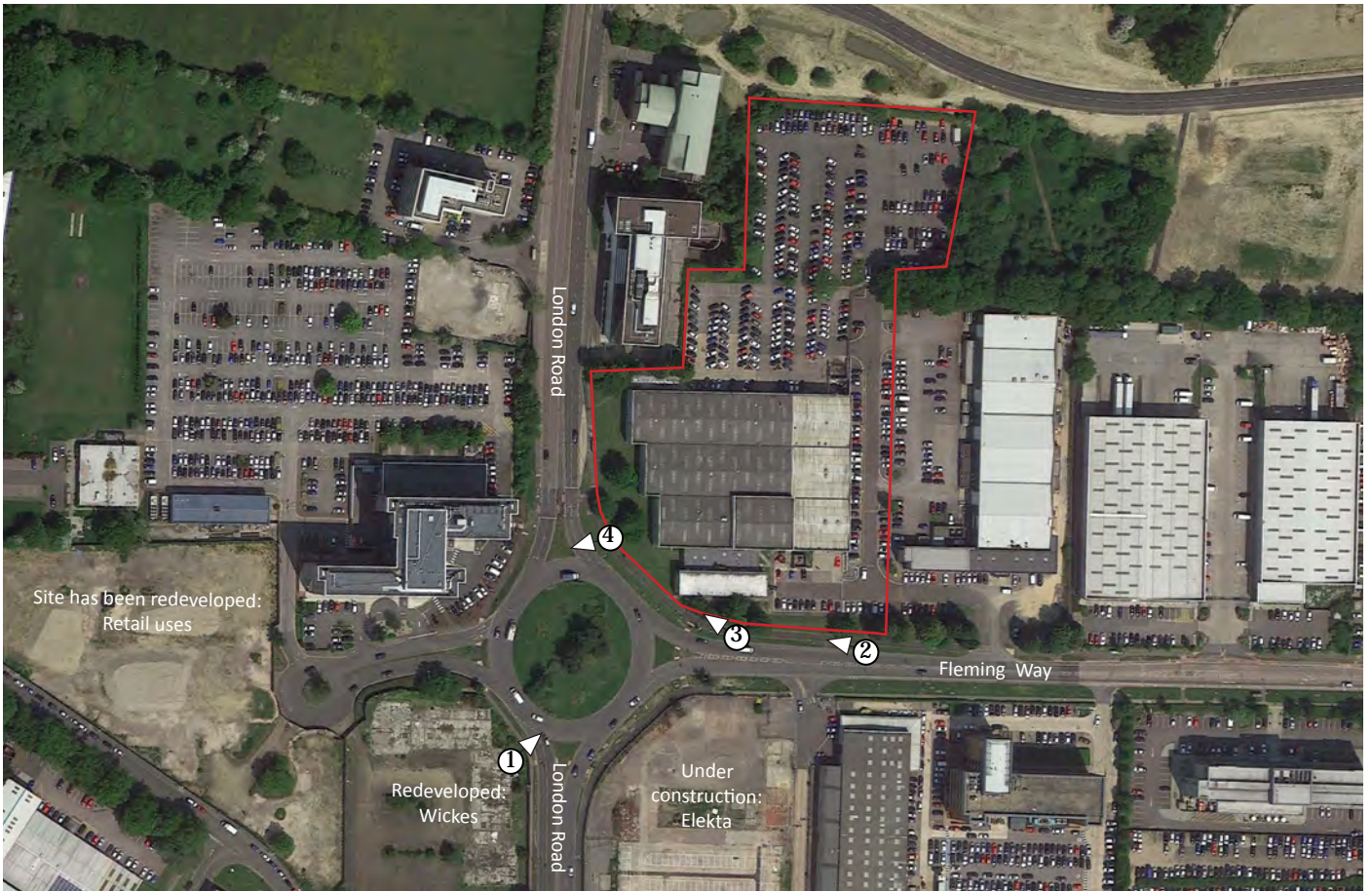
Aerial (Google Earth 2013)
