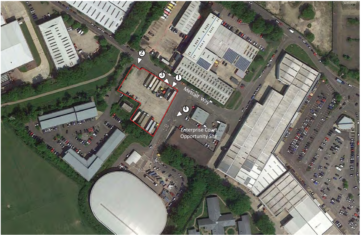
Aerial (Google Earth 2013)
