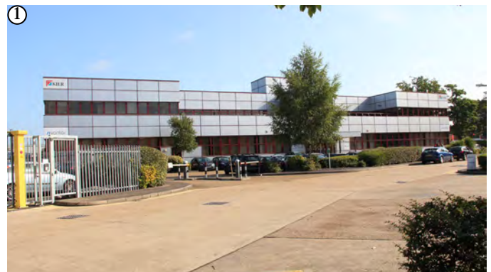
Office building located at the north-eastern corner of the site
