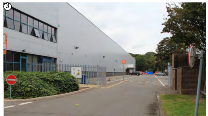
Parking area set back from Fleming Way frontage to the side of the existing building.
