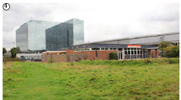
Single storey building close to southern boundary. Taller buildings (left) associated with Manor Royal Primary Gateway 3 (as defined in SPD)
