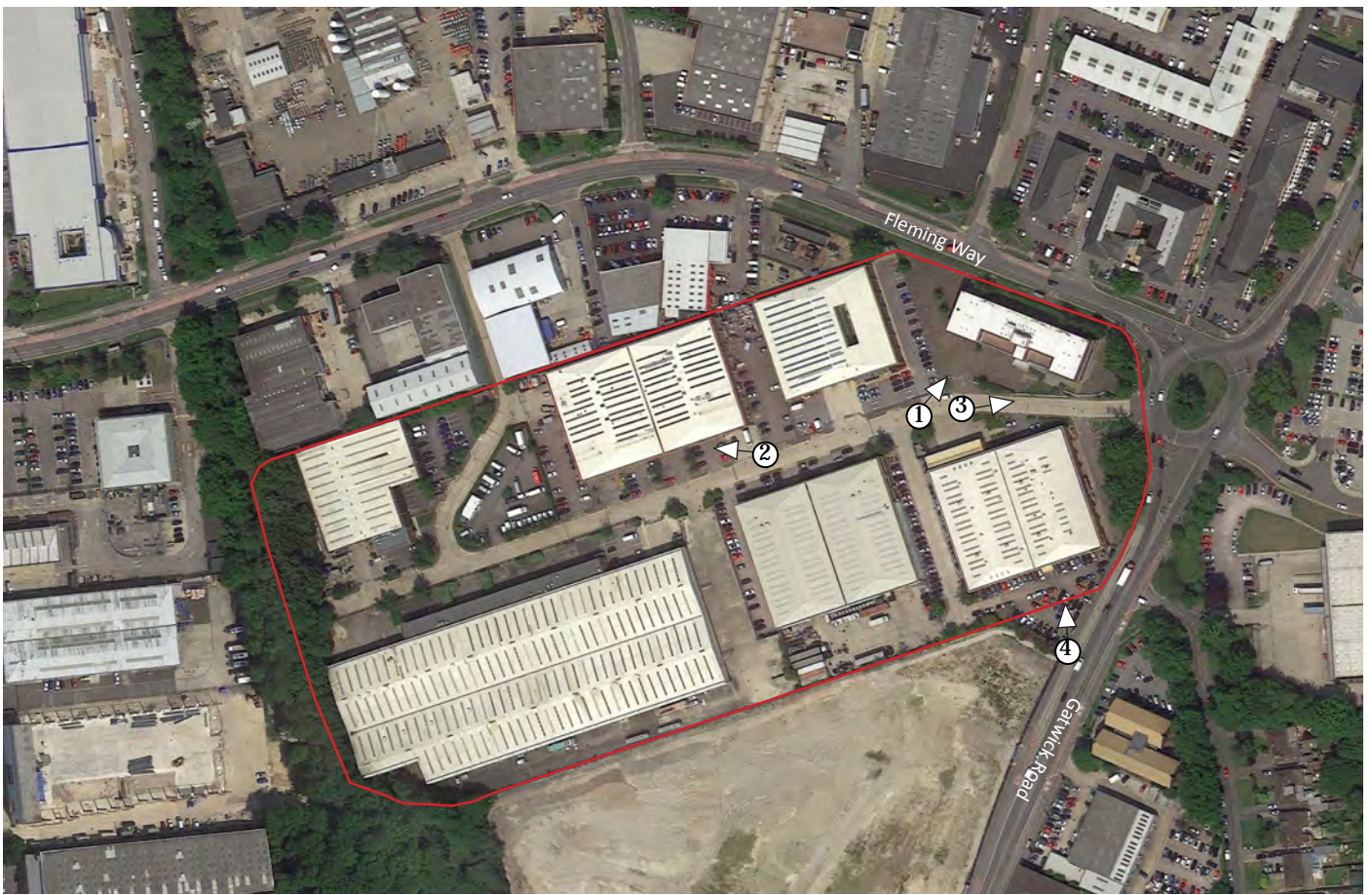
Aerial (Google Earth 2013)
