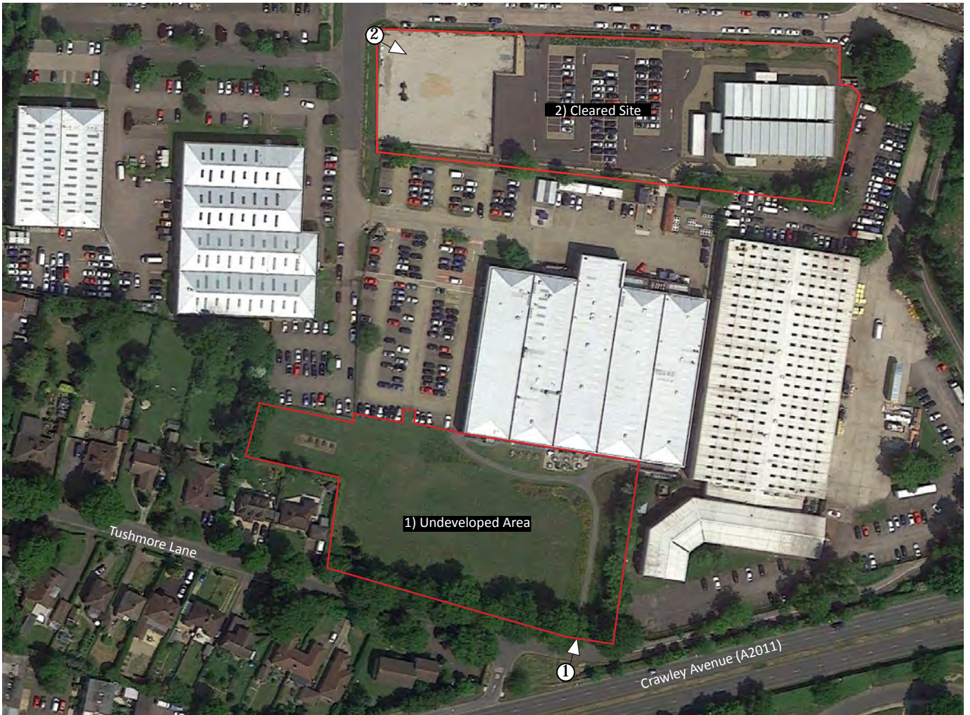
Aerial (Google Earth 2013)
