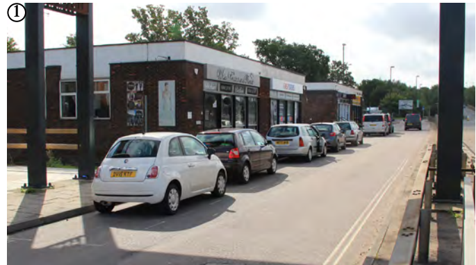
Existing single storey retail units
