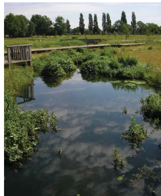
River Quaggy restoration and flood alleviation scheme, Sutcliffe Park, LB Lewisham, © Environment Agency
