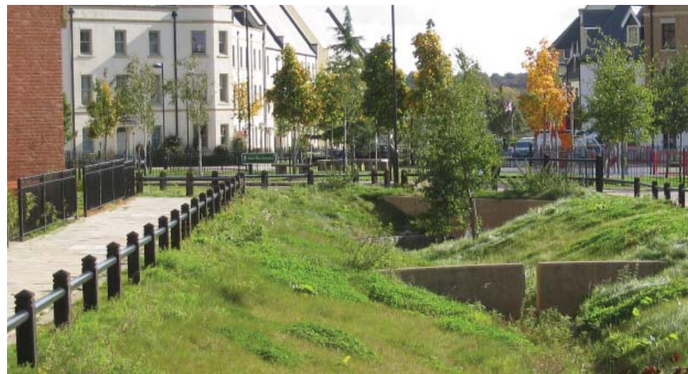
Swale forming part of SUDS at Upton eco-extension, Northampton, © Andy Gale
