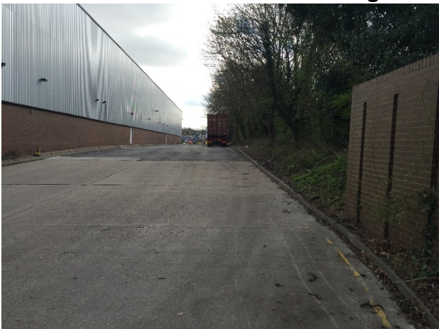
Location of existing surface water runoff into adjacent Eezehaul site
