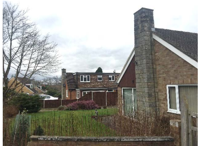
Example of stone work chimneys, Birch Lea
