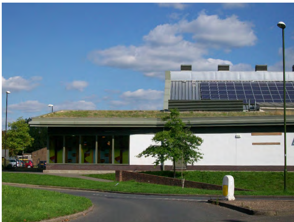
Figure 12: Green Roof at the Bewbush Centre
