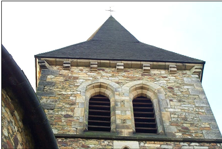
Figure 7. Details of stonework spire, Church of St. Nicholas'
