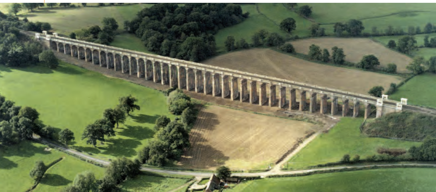
Ouse Valley Viaduct, Balcombe
