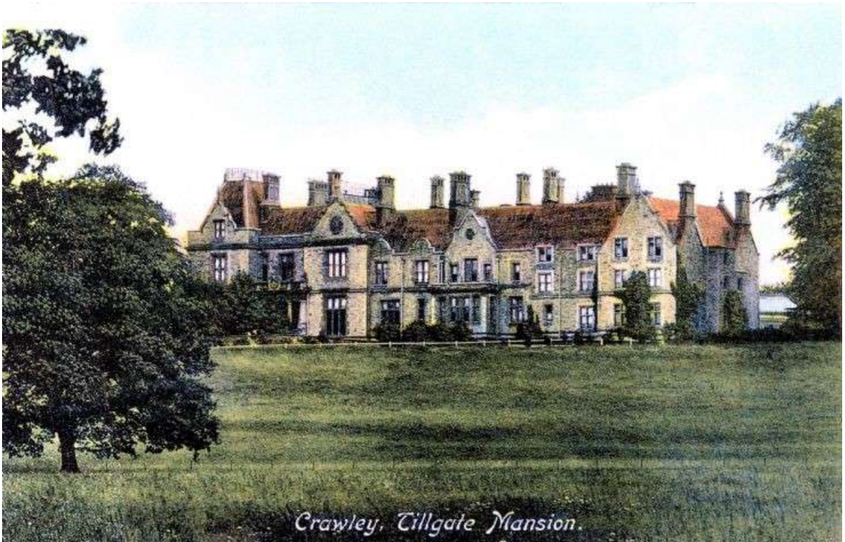
North front, Tilgate House, 1907
