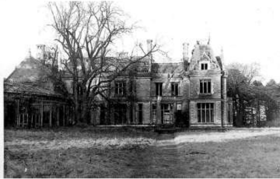
South front, Tilgate House, showing conservatory, c1960
