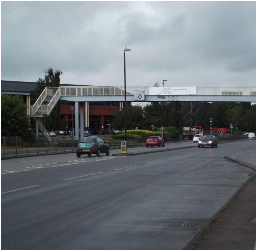
Figure 29: Existing approach to Manor Royal at Gateway 1
