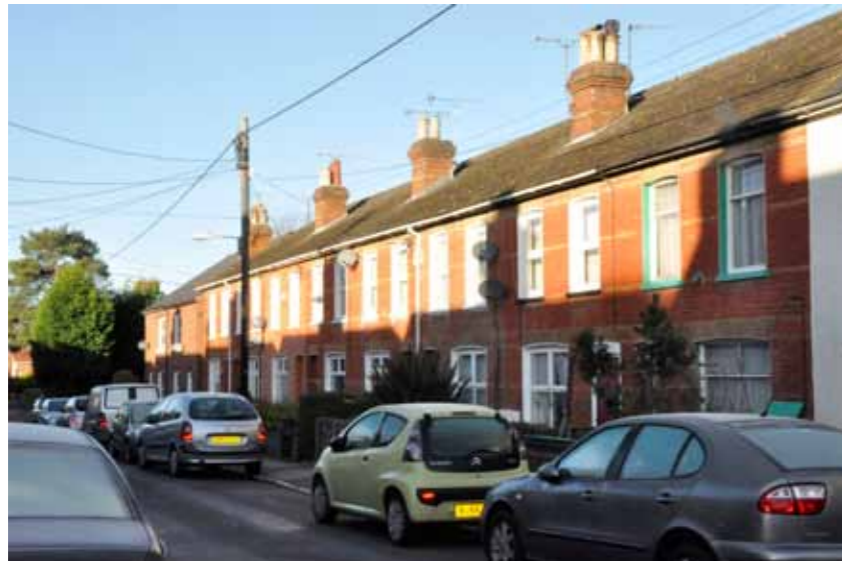
The terraces on the south side of the street have variegated brick but the quality of the architecture is unexceptional and the windows have been replaced with uPVC
