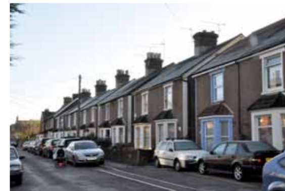
The character of the north side of the street has been eroded by replacement uPVC windows and concrete render
