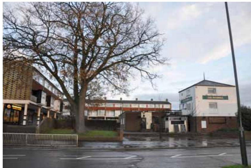
View of the pub and parade from across the street. The parade fronts the open space, which is well overlooked by the flats
