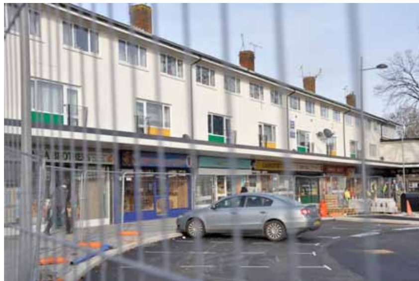
The shopping parade fronts the car park and a small green space. There are also some mature trees near the parade and on the green.
