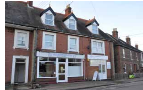
Historic shopfronts survive in some buildings
