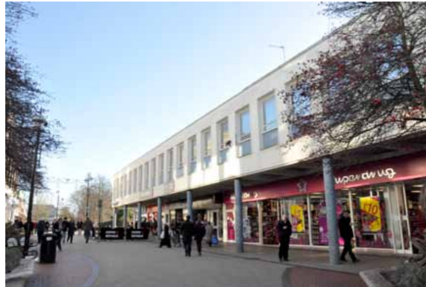
Tiled pilotis on Queensway
