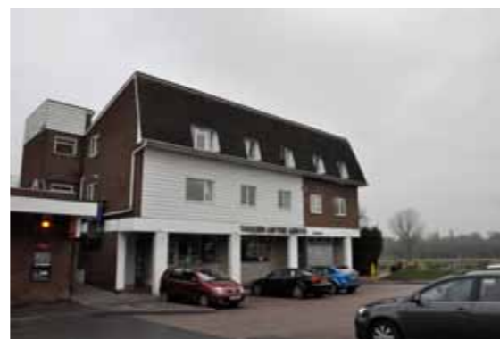
The pub is attached to the parade but differs markedly in height and architectural style.
