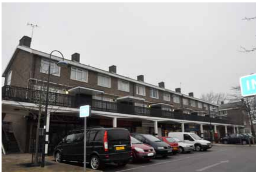
The parade and flats relate well to the public realm. Unlike other shopping parades in Crawley, flats in this instance are accessible from the front rather than the back. The shops' canopy is well integrated to the flat's entrance.
