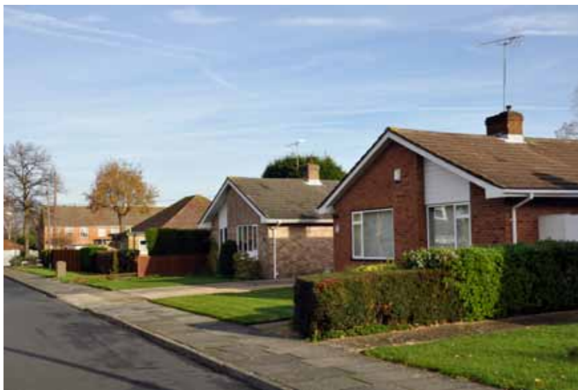
The one-storey bungalows located on Bracken Close do not present any urban, architectural or landscape feature of interest
