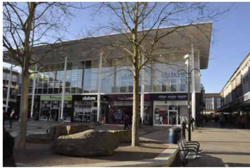
This infill building was constructed on Queen Square because it was originally too big
