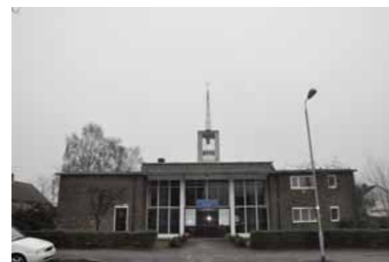
The Church/community centre has an attractive architectural composition.
