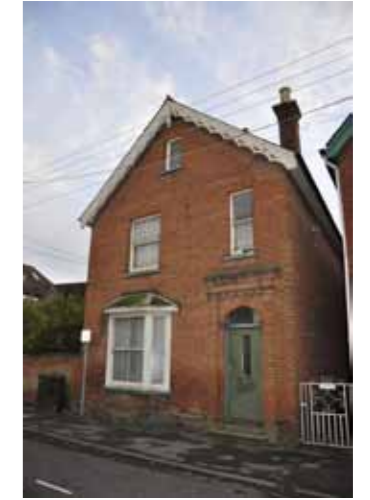
There are large well-preserved houses on Springfield Road with decorative barge boards, original sash windows and decorative brickwork
