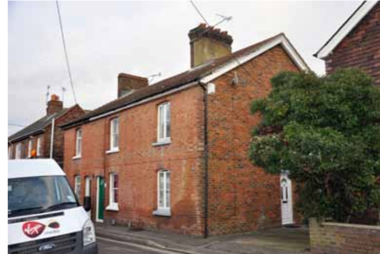
The buildings are modest but of pleasing proportions with variegated brickwork
