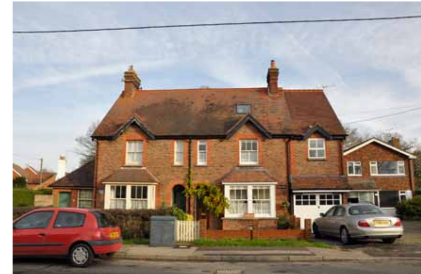
The majority of buildings on Ilfield Green are Victorian or Edwardian and well-presented
