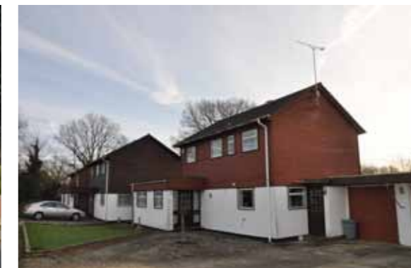
It seems likely that these weatherboarded houses on the south side of the Lane were built by the Development Corporation
