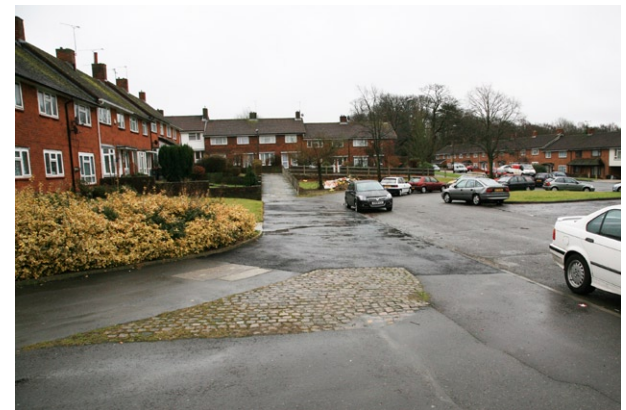
Poor quality amenity spaces, parking and public realm in Gossops Green.
