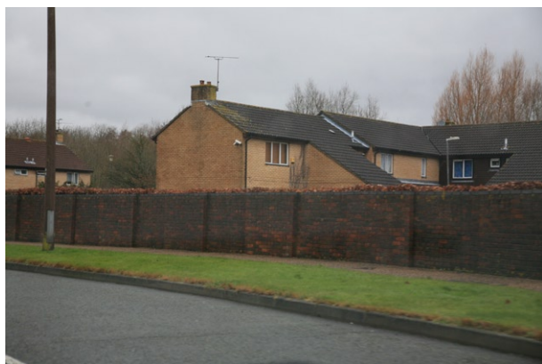
Rear fences creating a poor quality street environment, Bewbush
