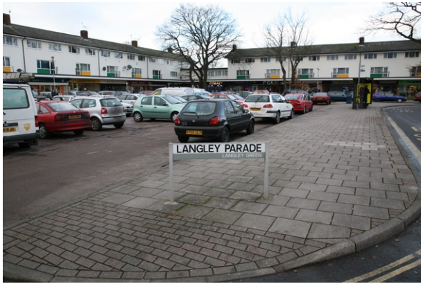
Car parking dominating the neighbourhood centre at Langley Parade, Langley Green.
