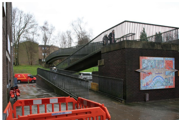
Poor quality public realm and pedestrian access bridges at Broadfield neighbourhood centre.
