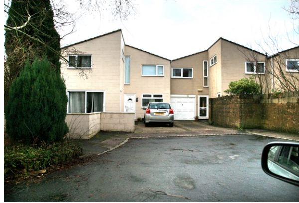
IMG_3584 Laurel Close Furnace Green
