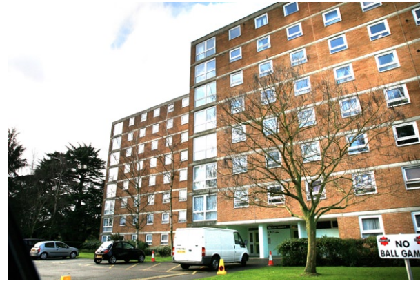
IMG_3913 Milton Mount Avenue Pound Hill North
