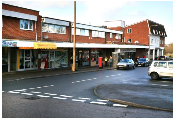
IMG_3876 Grattons Drive Pound Hill North
