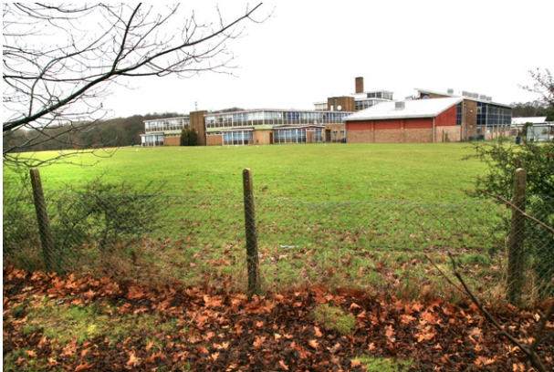
IMG_3425 Bewbush Drive near Admiral Road Gossops Green
