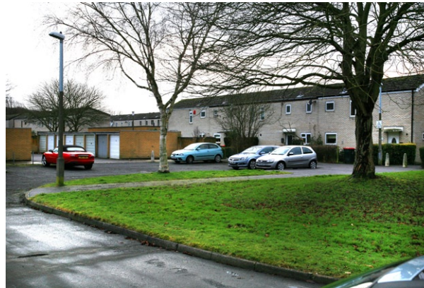
IMG_3613 Norwich Road Furnace Green
