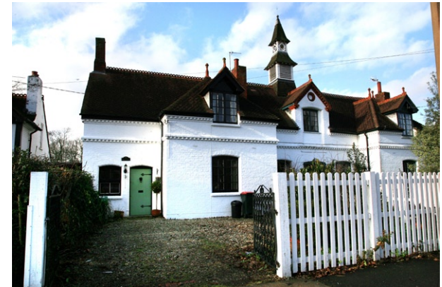
IMG_3871 Grattons Drive Pound Hill North
