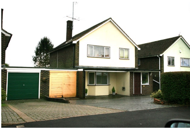
IMG_3618 The Glade Furnace Green
