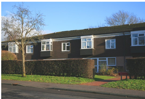
IMG_4014 Crossways / Hermits Road Three Bridges
