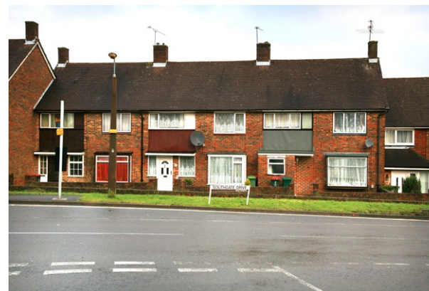
IMG_3670 Southgate Drive / Baker Close Southgate
