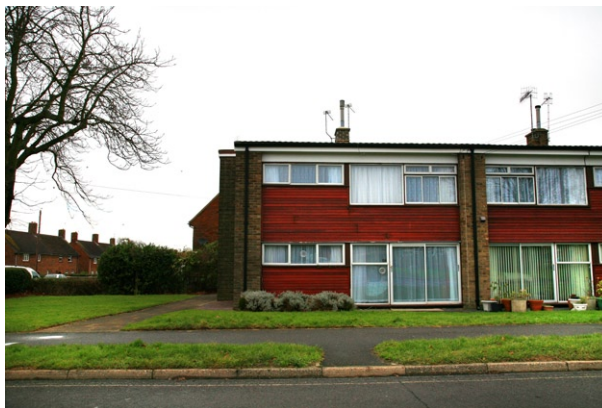
IMG_3010 Ewhurst Road near Ginhams Road West Green
