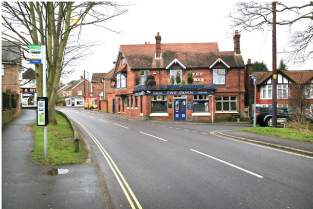
IMG_3066 Horsham Road / Church Street West Green
