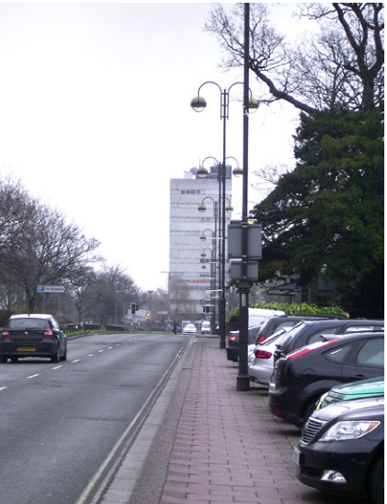
IMG_0227 View east along The Boulevard
