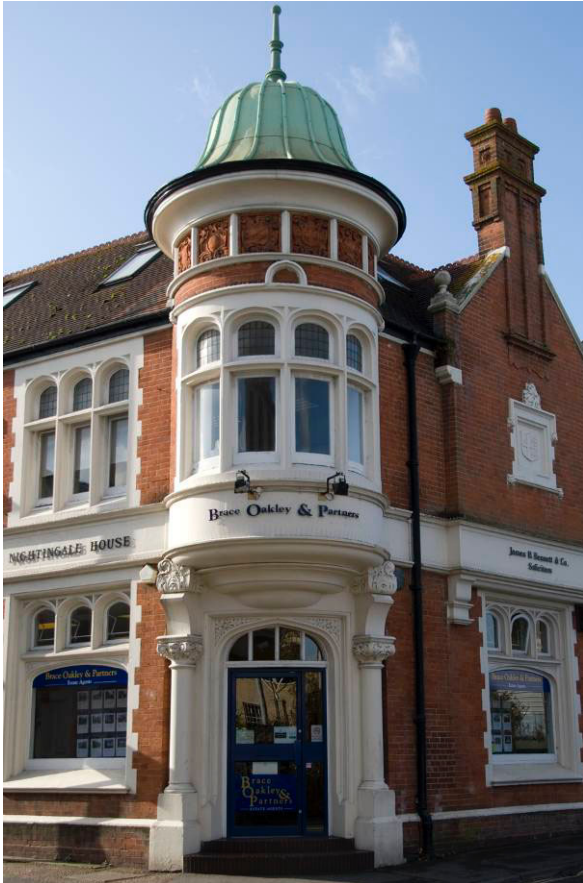
Fig. 22. Former London & County bank, Brighton Road.
