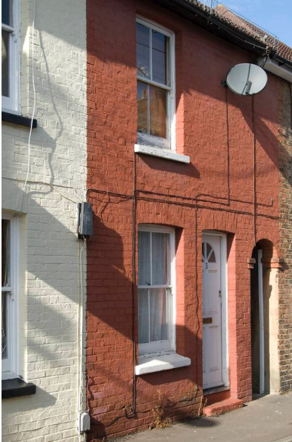
Fig. 20. Late 19 th -century terraced housing, West Street.
