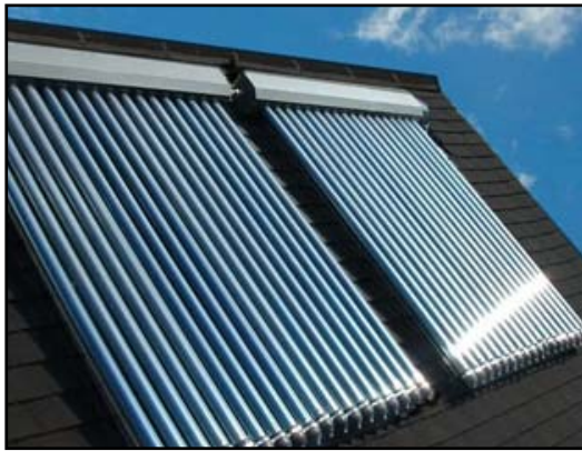
Figure 5: Evacuated tube collectors ( www.metaefficient.com )
