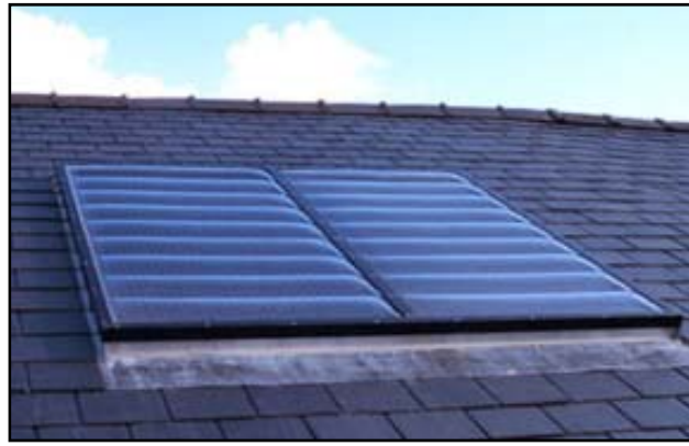
Figure 6: Flat plate collectors ( www.cat.org.uk )
