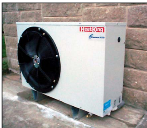
Figure 8: Air Source Heat Pump ( www.solheat.co.uk )
