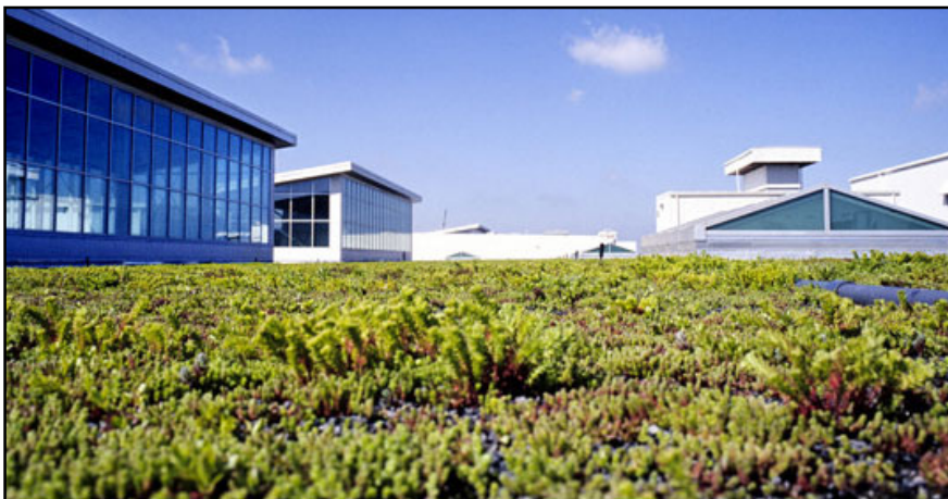
Figure 14: A green roof ( www.inhabitat.com )
