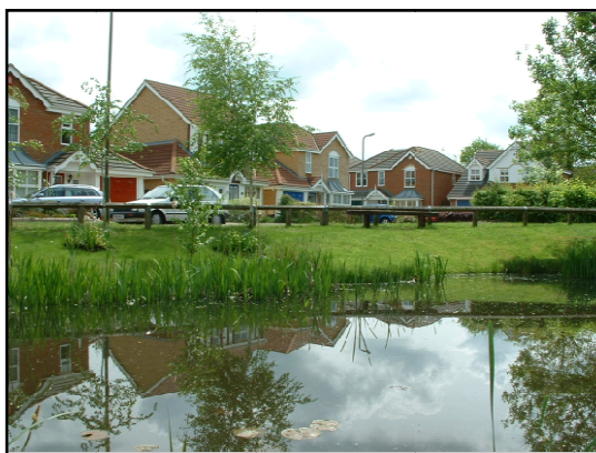
Figure 13: Balancing ponds at Holmes Close, Woking. These also act as an amenity asset. (Woking BC).
