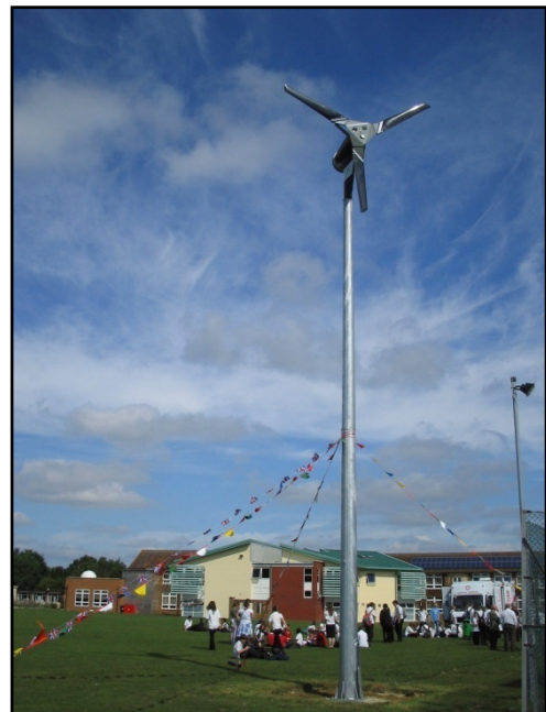
Figure 3: A 2.5kW wind turbine at Ringmer Community College, East Sussex (ecsc)
