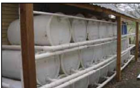
Figure 16: Linked rain barrels storing rain water ( www.harvesth2o.com )
