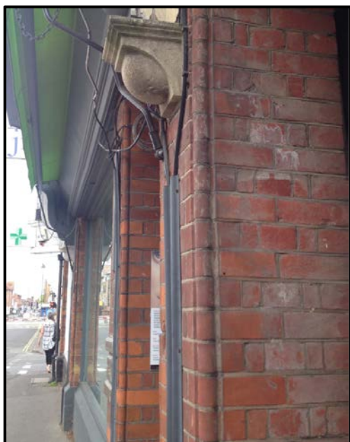
Figure 3.8. Brickwork at no. 16 Brighton Road, taken August 2017
