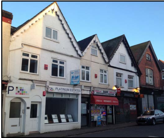
Figure 3.21. Shop fronts at nos. 6-12 Brighton Road, taken March 2018
