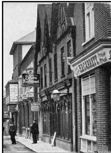
Figure A1.9. Shop fronts on eastern side of Brighton Road, c.1905
