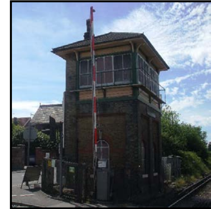
Figure A1.8. Signal box, June 2014
