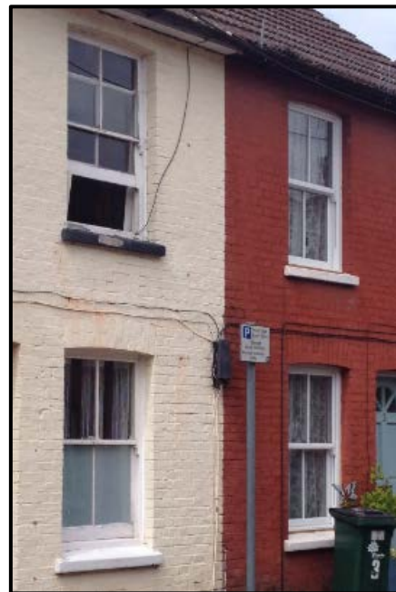
Figure 3.29. Preserved sash windows at nos. 3-5 West Street, taken August 2017
