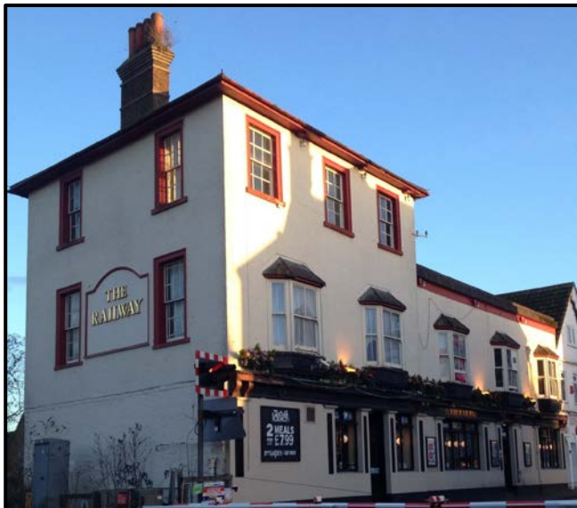
Figure 3.7. The Railway Hotel, taken March 2018
