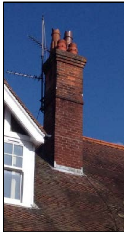
Figure 3.11. Roof detail and chimney at no. 14 Brighton Road, taken August 2017
