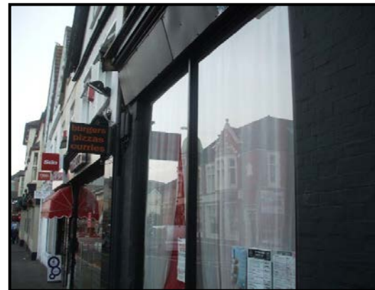
Figure A1.10. Shop fronts on eastern side of Brighton Road, September 2014
