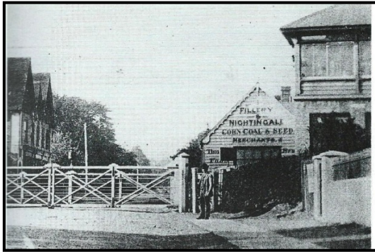
Figure A1.6. Level crossing and signal box viewed from the north, late 19 th century
