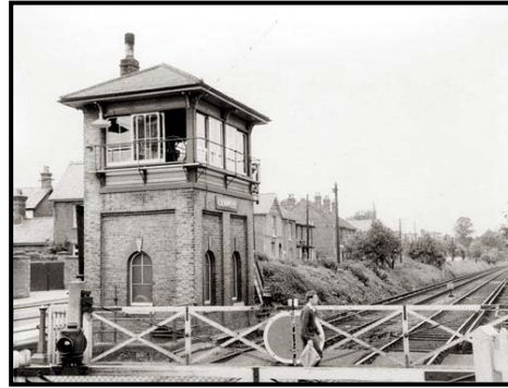
Figure A1.7. Level crossing and signal box viewed from the south, c.1965
