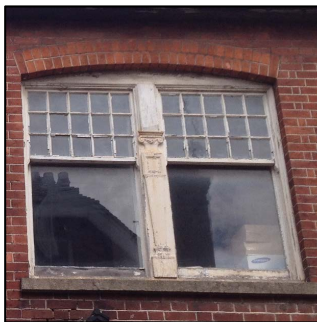
Figure 3.9. Original first-floor sash window at no. 12 Brighton Road, taken August 2017
