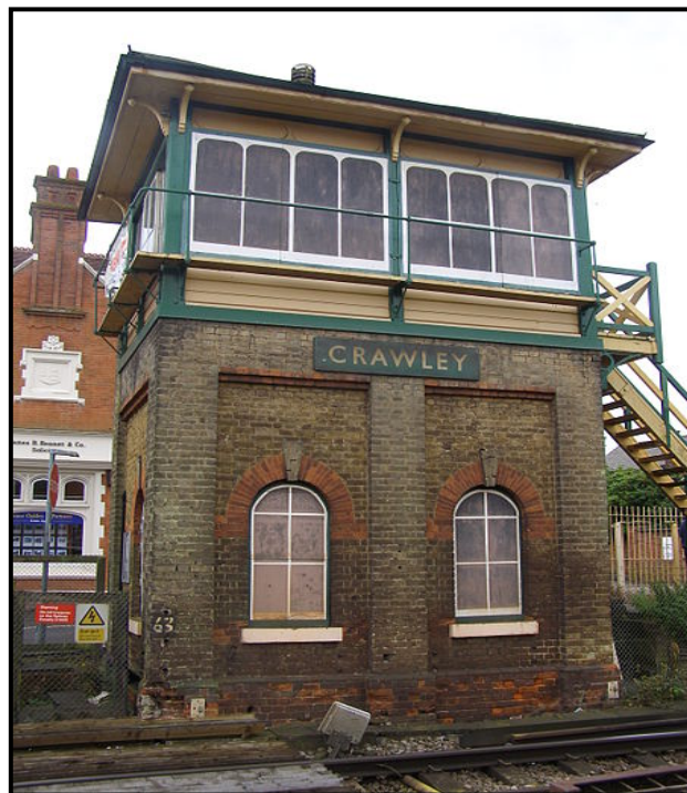
Figure 3.12. Grade II listed railway signal box
