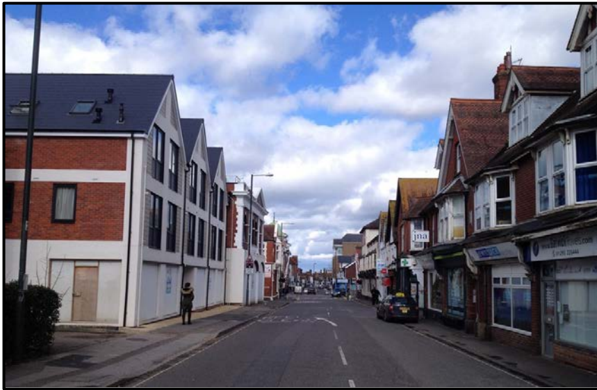
Figure 3.2. View 2: Northwards along Brighton Road from the southern end of the Conservation Area, taken March 2018
