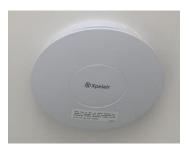
An extractor fan is fitted in the bathroom, this is set at a low fan rate that will increase when moisture levels increase. Do not turn this off.
