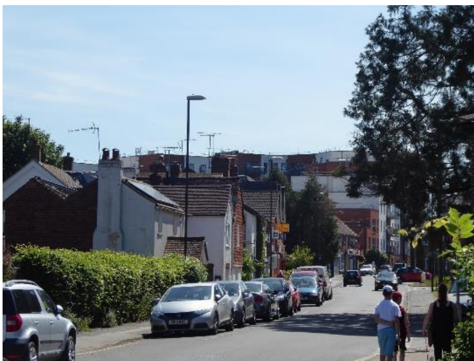
Figure 46 The view east through the Conservation Area, with recent developments dominating the view.
