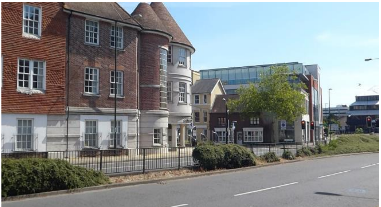
Figure 88 View East, toward the southern edge of the Conservation Area from Haslett Avenue West
