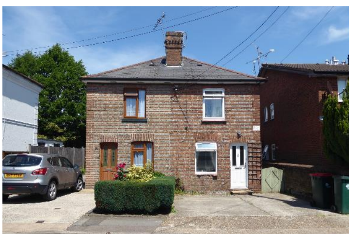
Figure 37 13 and 15 New Street
