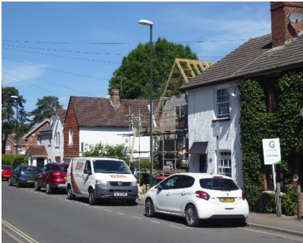
Figure 51 The new extension under construction on Ifield road looking west
