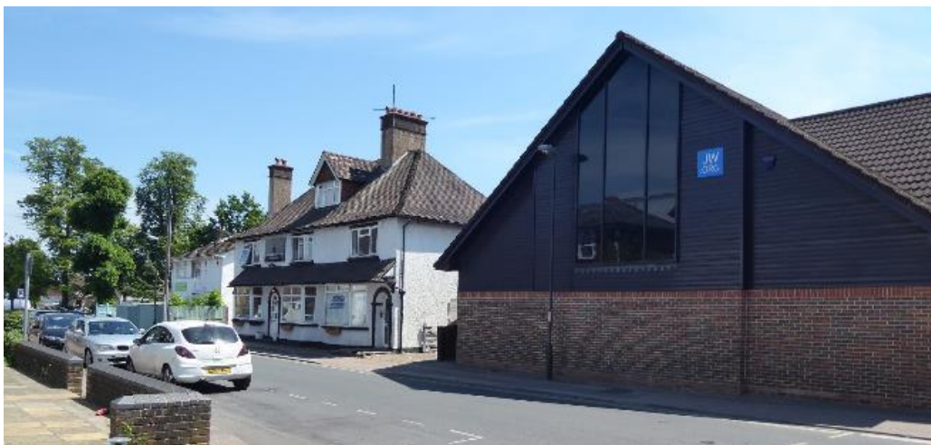
Figure 41 Three Bridges Road, south side
