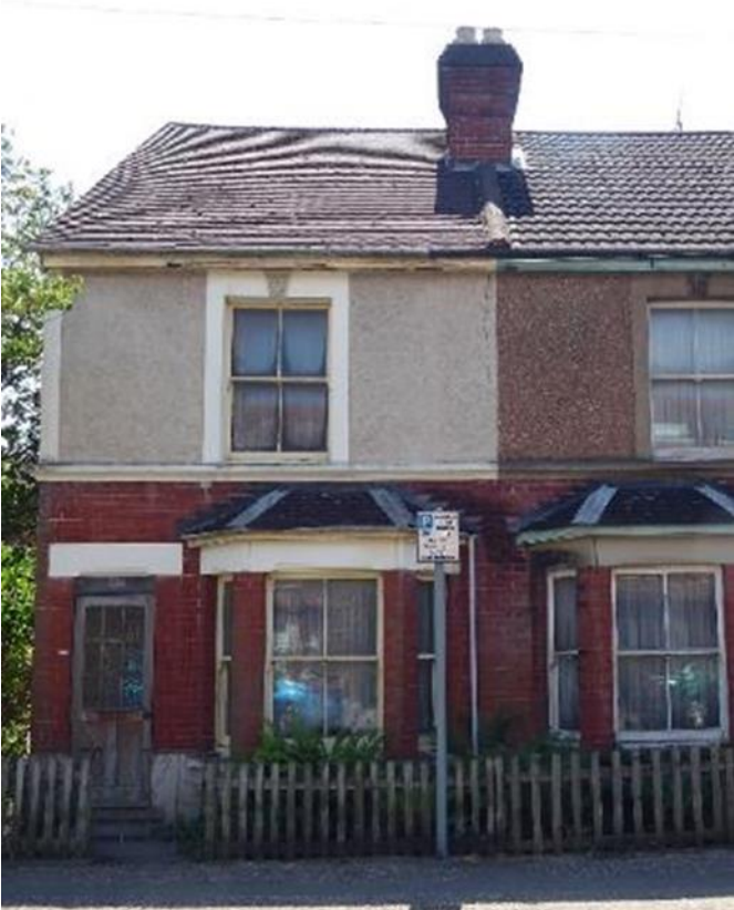
Figure 27 Original timber windows remain on some properties
