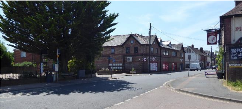
Figure 40 Three Bridges Road, looking west
