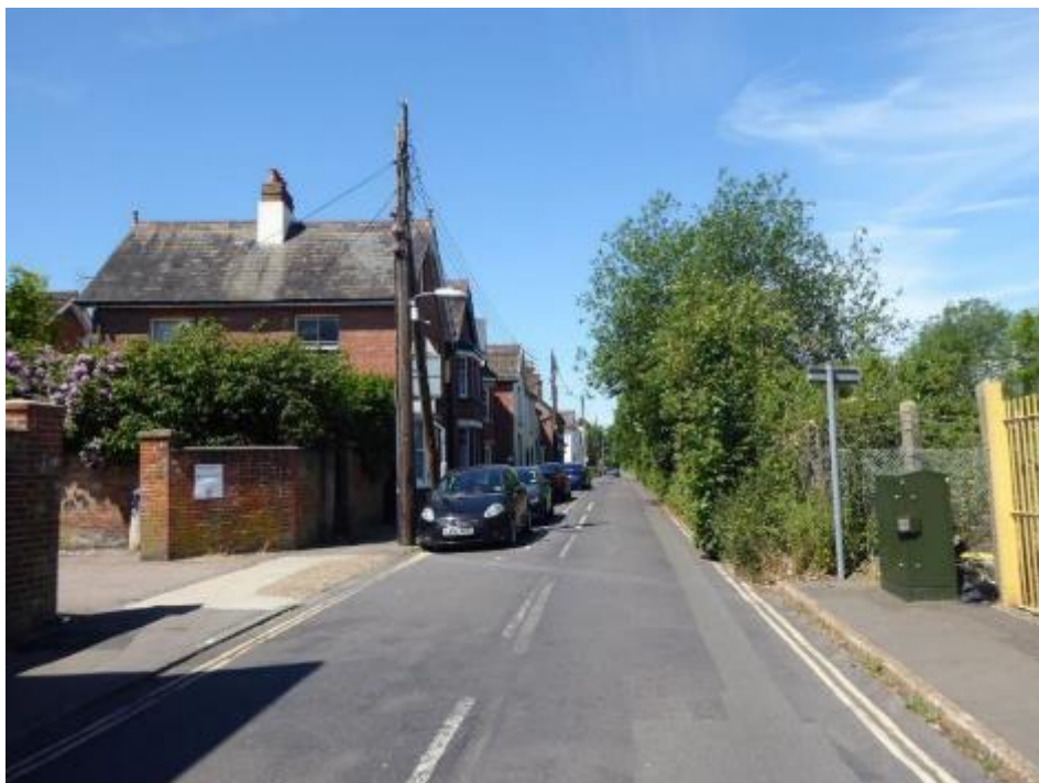
Figure 19 Viewpoint 2: The view within the Conservation Area west along Springfield Road from the Listed signal box.
