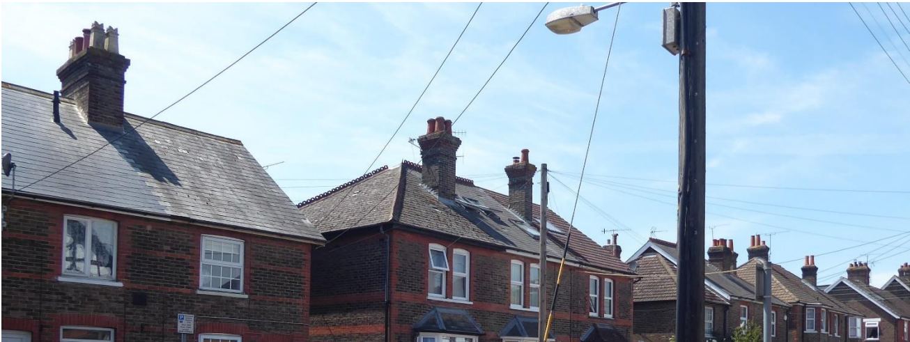
Figure 24 Breaks in built form and through roads are representative of the original development plan, preventing built form from being overbearing
