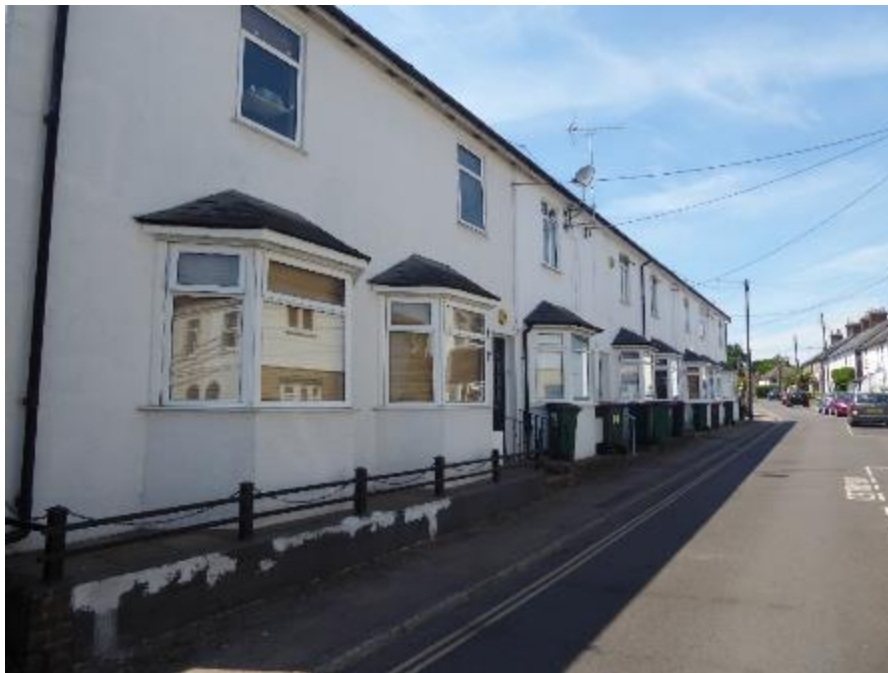
Figure 30 Terraced Houses on New Street (south side). Heavily altered, these houses do not display the architectural features which contribute to the significance of Hazelwick Road
