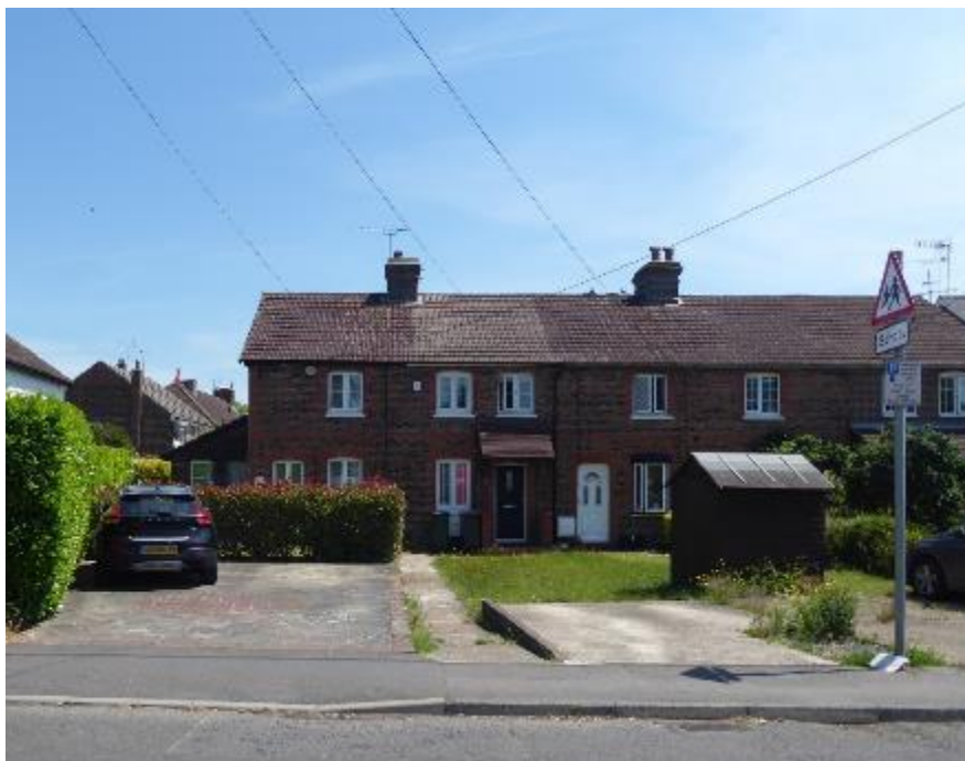
Figure 29 Nineteenth century cottages on North Road, east side, which feature uPVC windows, unsympathetic porches and doors
