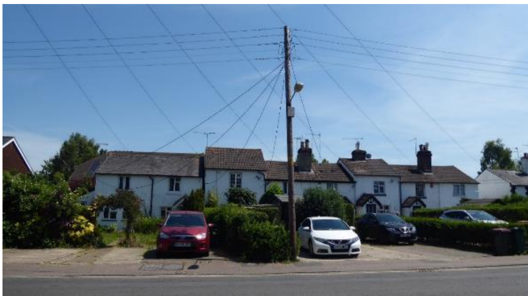
Figure 31 Locally Listed terrace on North Road
