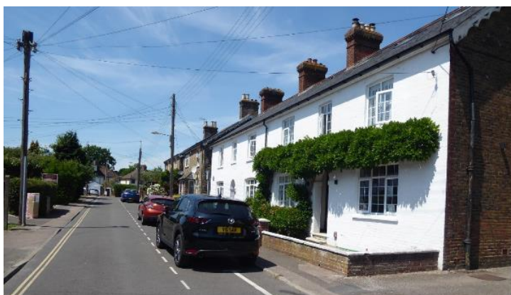
Figure 36 51 and 53 New Street
