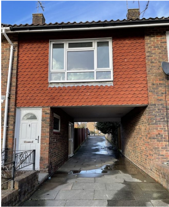
Figure 6. Covered footway, Rother Crescent
