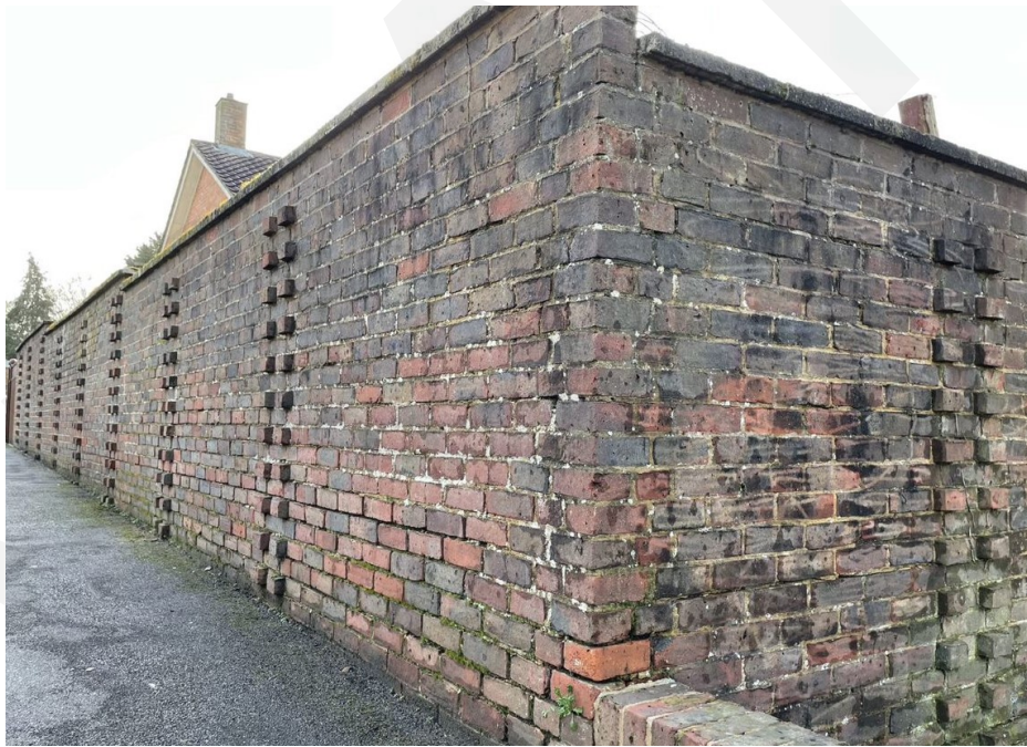
Figure 3. Detailing on a brick boundary wall on Medway Road
