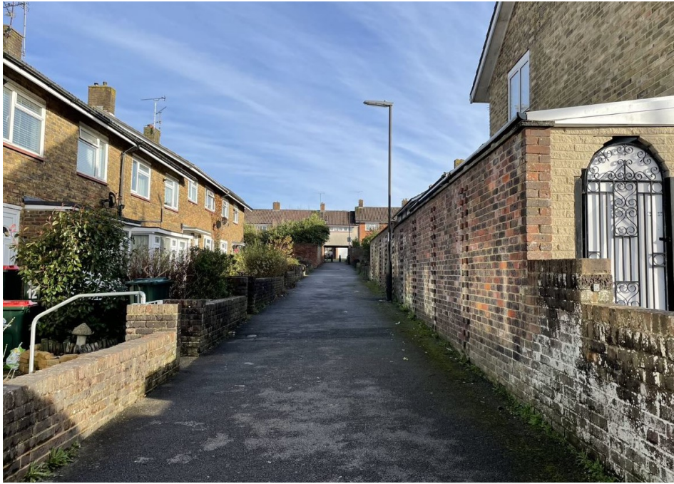
Figure 2. Varieties of brickwork on a walkway in Lavant Close
