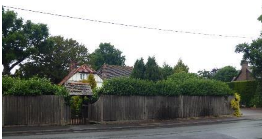
Figure 51 Turks Croft, a Grade II listed building. The older rendered range is largely concealed from the street scene
