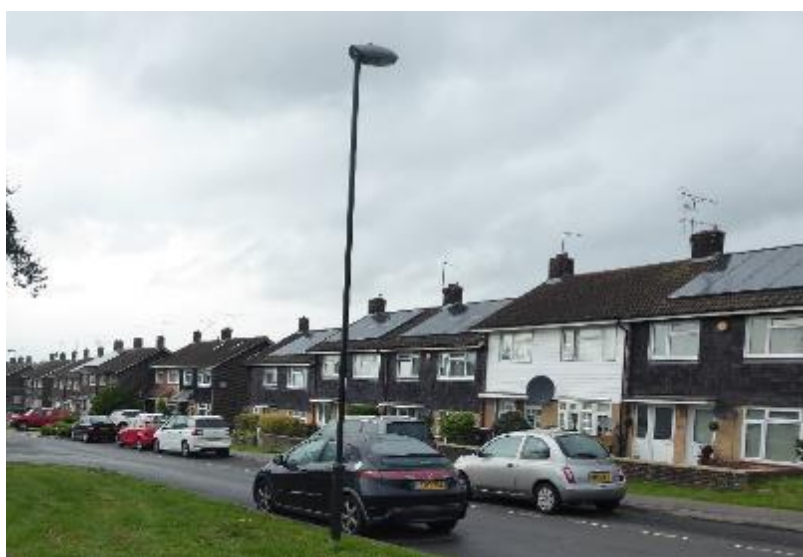
Figure 26 Terraced houses on Medway Road, opposite St Albans Church, satellite dishes, solar panels and alterations to cladding, windows and porches dilute the homogeneity of the area
