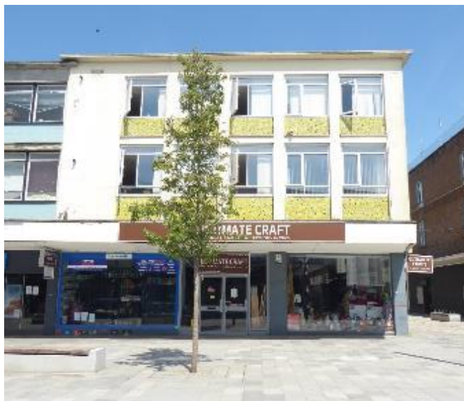
Figure 38 Mosaic tiles and inappropriate signage, located on the canopy
