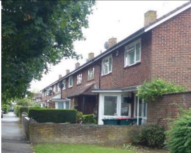
Figure 47 The loss of original porches (centre) detracts from the street scene
