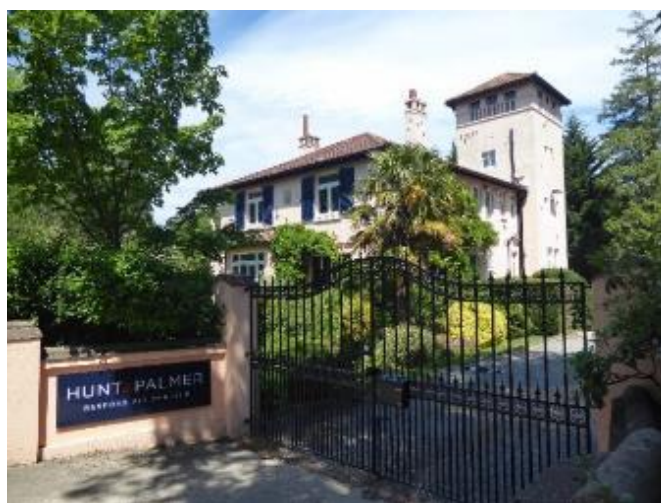
Figure 22 Masons Hall (formerly Goffs Tower)
