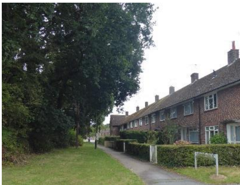
Figure 49 Boundary Close, perpendicular to the main road, has a secluded, quiet appearance, with parking located to the rear
