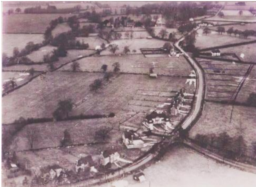
Figure 38 Aerial view of Rusper Road taken in the 1930s ( http://iansapps.co.uk/oldbritain/crawley/rr.html )
