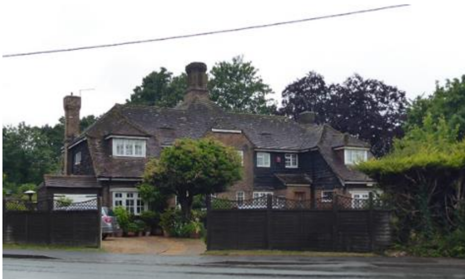
Figure 39 Cat slide roofs, dormer windows and timber boarding, typical of the Arts and Crafts style of the ASLC
