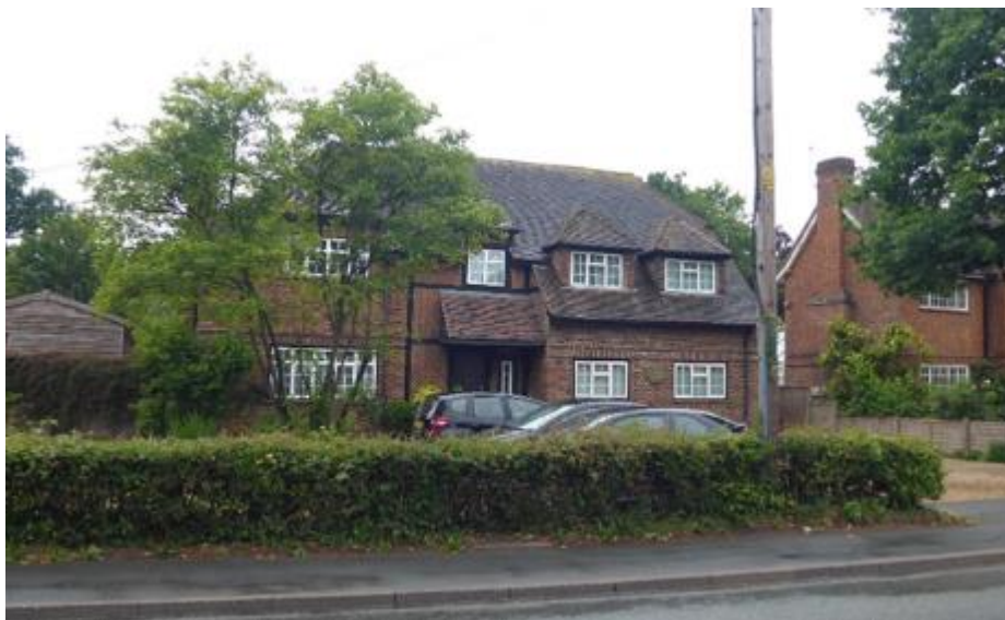
Figure 40 Dormer windows, exposed timber beams and decorative brickwork feature on all the houses (excluding Le Chantier)
