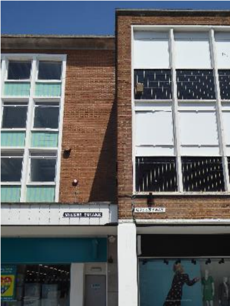
Figure 45 Window Aprons in sheet metal and original street signs, Queensway
