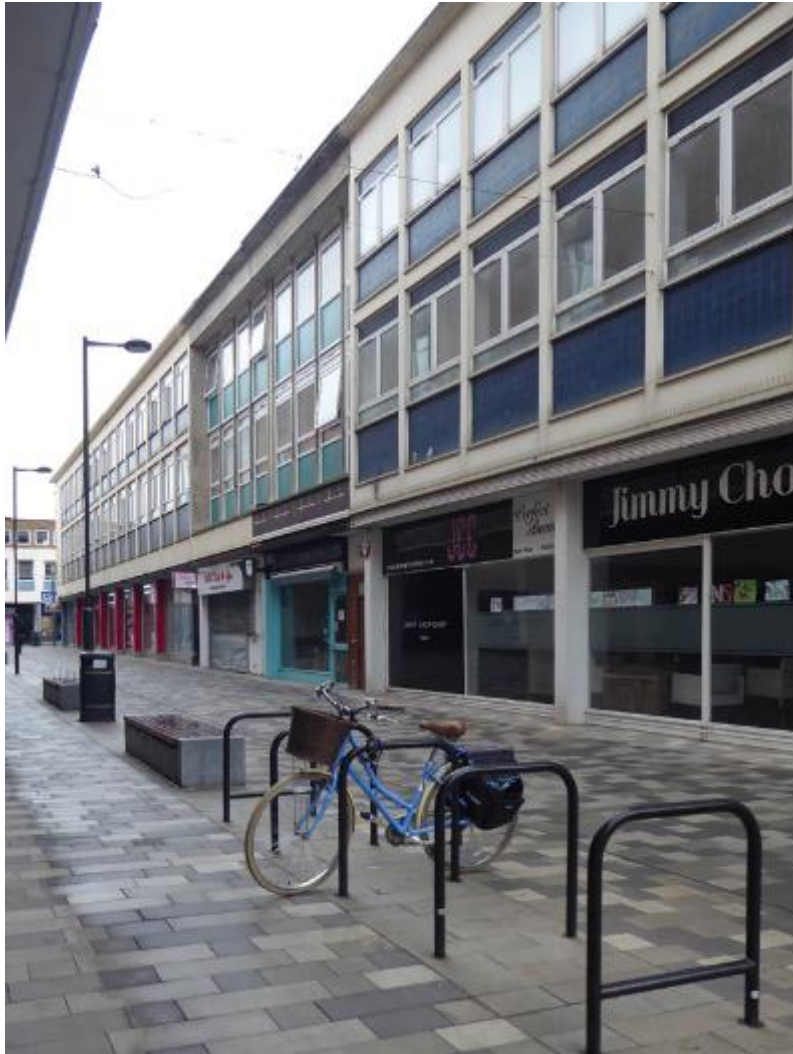
Figure 46 Buildings are constructed in a modular formation, retail space correlating to the bays and fenestration on higher floors, The Pavement, looking south
