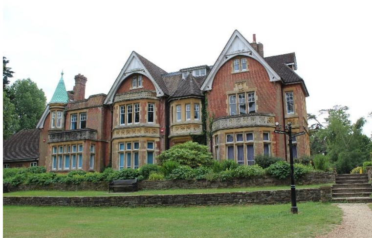
Figure 5 View south towards Goffs Park House and raised border planting
