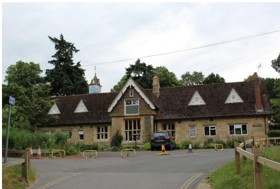
Figure 22 Former stable block
