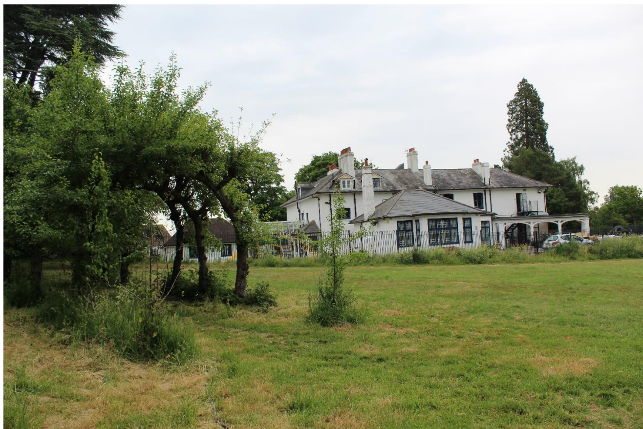
Figure 3 View north of arbour and Broadfield House
