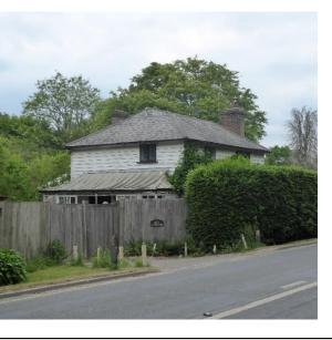
Ten sixty-six has red stock brick at ground floor with white timber weatherboarding at first floor. The roof is of slate. The leaded windows at ground floor level appear to be original. To the south elevation is a veranda with a swept rolled lead roof, enclosed partly with glazing.
